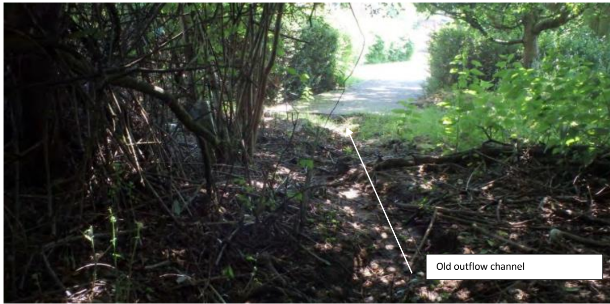
Figure 17, View from Outflow Channel Looking South Down the Access Path. Photo from Lidar Logic, September 2021.
